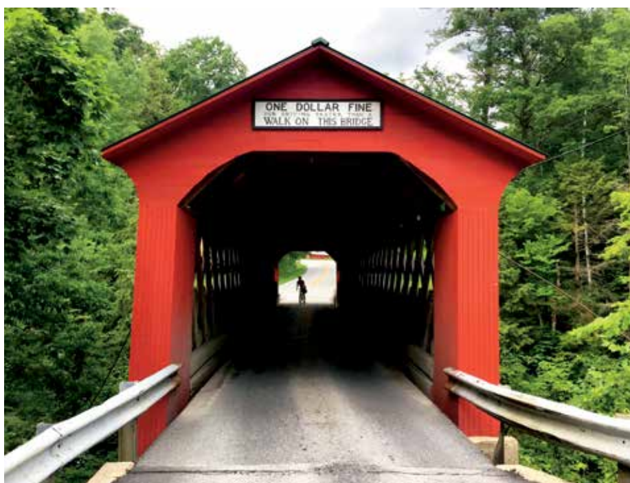
Chiselsville Covered Bridge, East Arlington, Vt.
